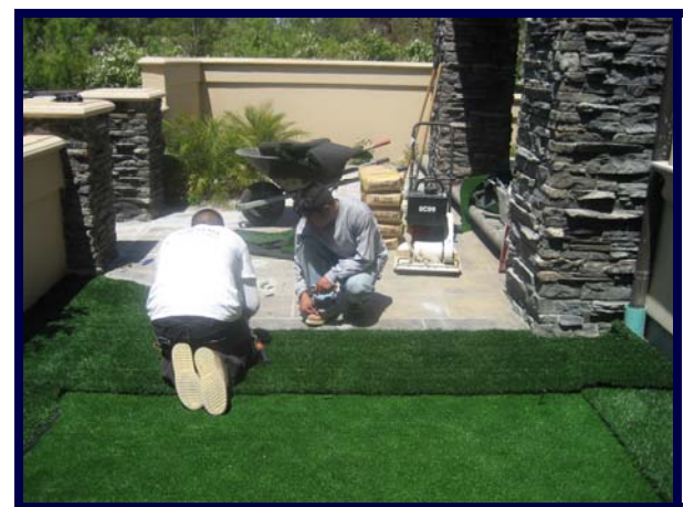
Lay the lawn turf on the border area and trim to fit. Take your time and be accurate!
