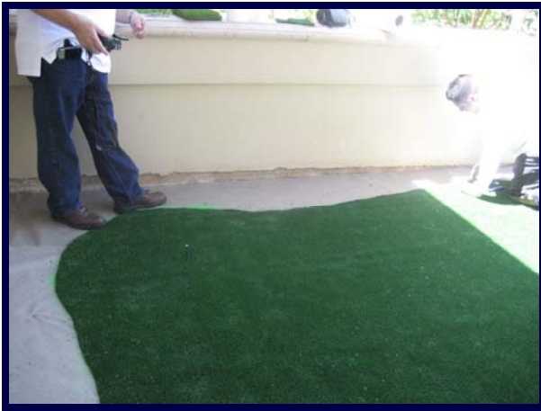
Trim to the masking tape lines and join the pieces with seam tape and PL400 Liquid Nail adhesive.
