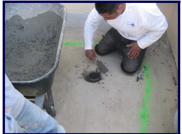
Place the cup in the hole and secure with cement.
