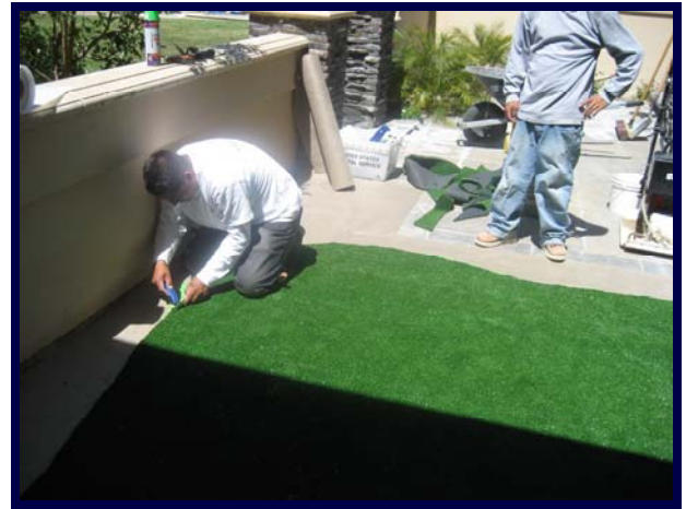
Trim to the masking tape lines and join the pieces with seam tape and PL400 Liquid Nail adhesive.
