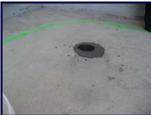
Level with sub-base.
