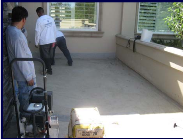
Lay down the sub-base and compact it to 95%
