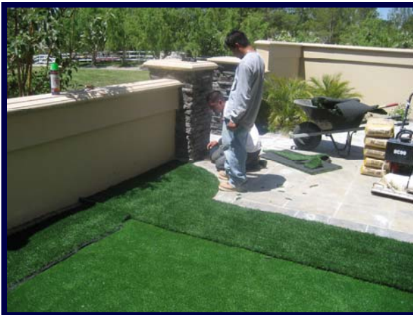
Lay the lawn turf on the border area and trim to fit. Take your time and be accurate!
