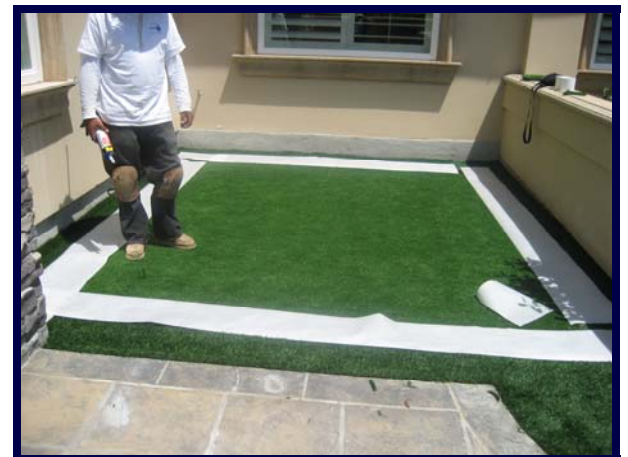
Lay down Seam tape on top of all the seams and trim to length.
