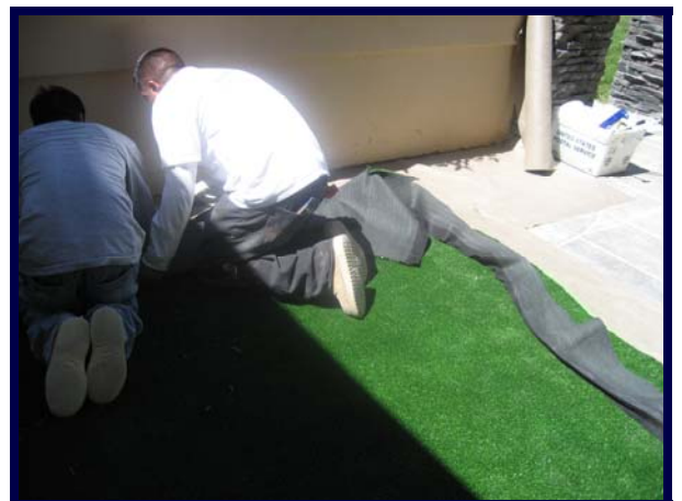
Lay down the turf, starting in one corner.
